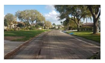
There is some debris left in the roadway and the pavement is uneven so PLEASE be very safe in this area. The debris will affect the friction course and you will not have the same stopping power you had with the original roadway.
